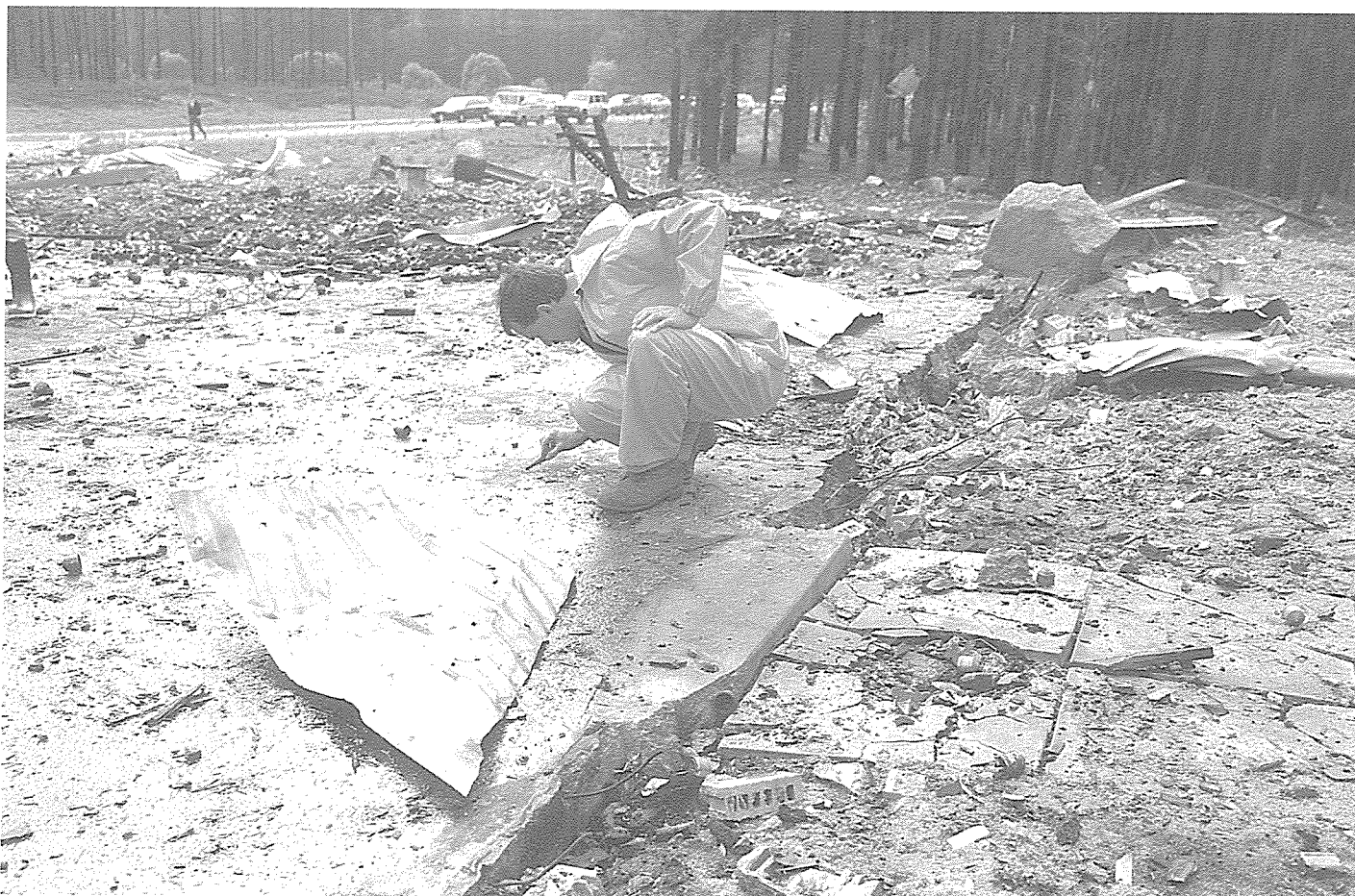
Henry Zuidersma of our Explosives and Dangerous Goods Division inspects the site of a deliberate explosion at the Baldivis Explosives Reserve which destroyed a magazine and was heard up to 25 kilometres away.
