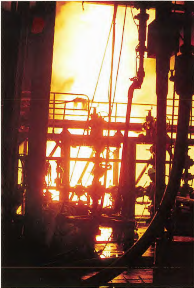
Drill floor view of well-test flare during development of the Harriet Field.
