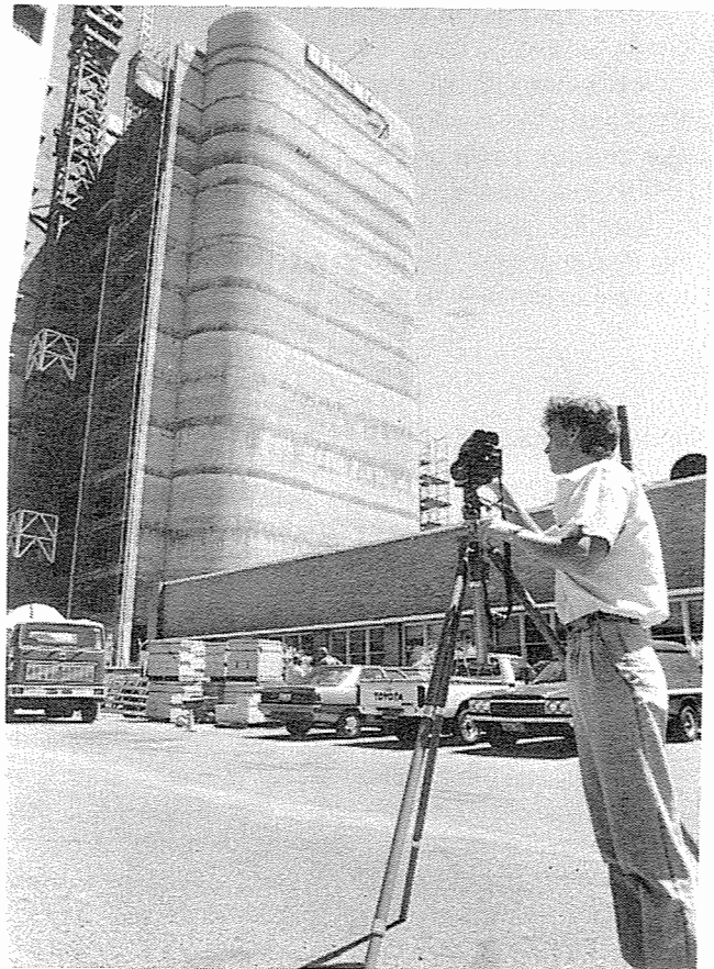
Photographically recording progress on construction of Mineral House Stage 2.
