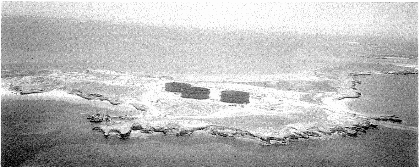
Varanus Island in the Lowendal Group showing storage tanks of the terminal for the offshore Harriet oilfield.
