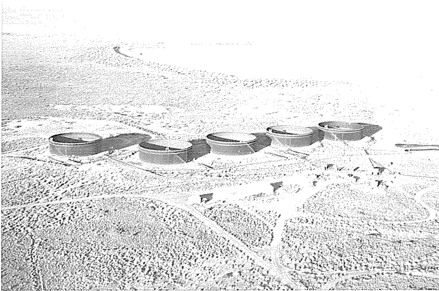
Oil Storage tanks at Barrow Island (WAPET photo).
