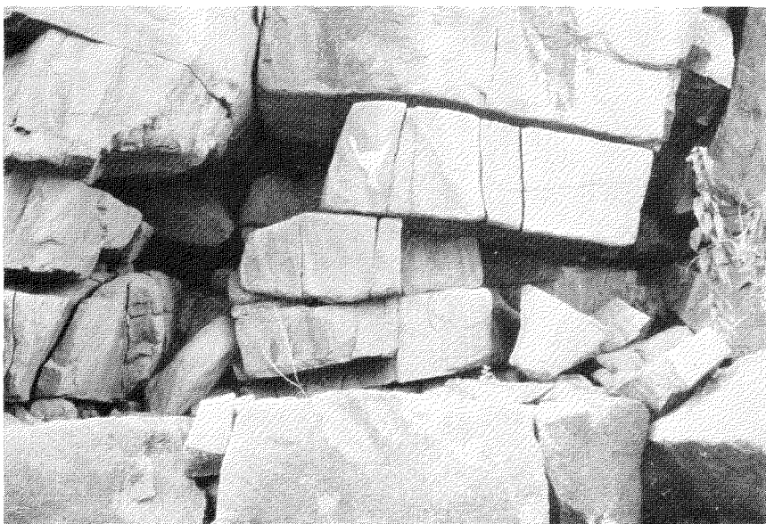
C. Hillside Dam Site, large joint openings in the dolerite; F1192.
