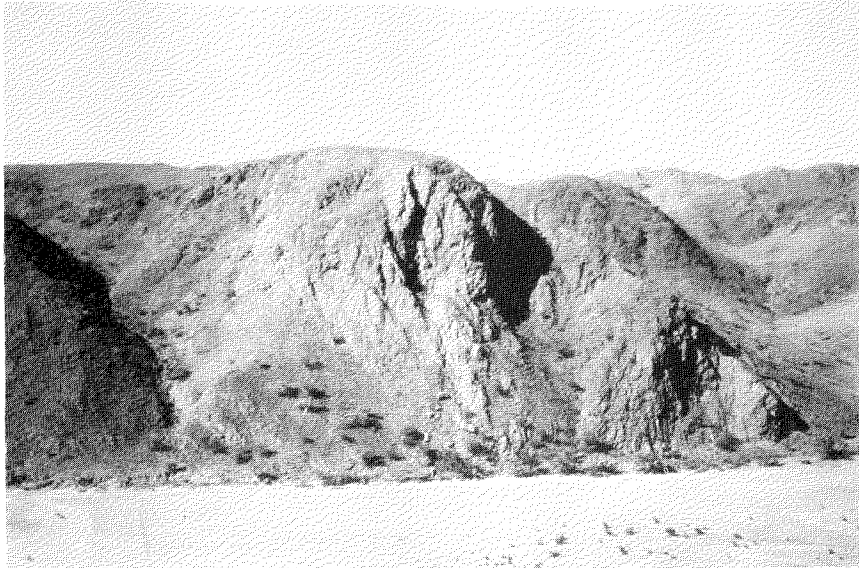
A. North Pole Dam Site, right abutment viewed from left abutment; F1190.
