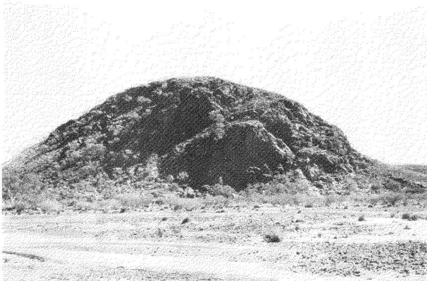
B. North Shaw Dam Site, the anticlinal folding forming the left abutment, and the faulting and large joint openings are shown; F1191.
