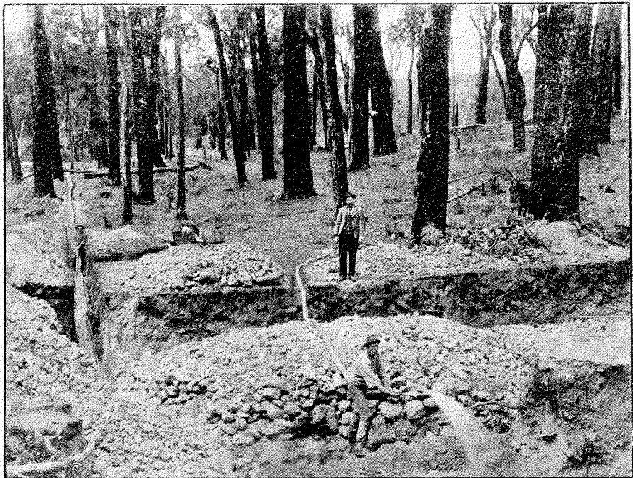
Westralian Tinfields, Ltd., Hydraulic Sluicing, Greenbushes.
