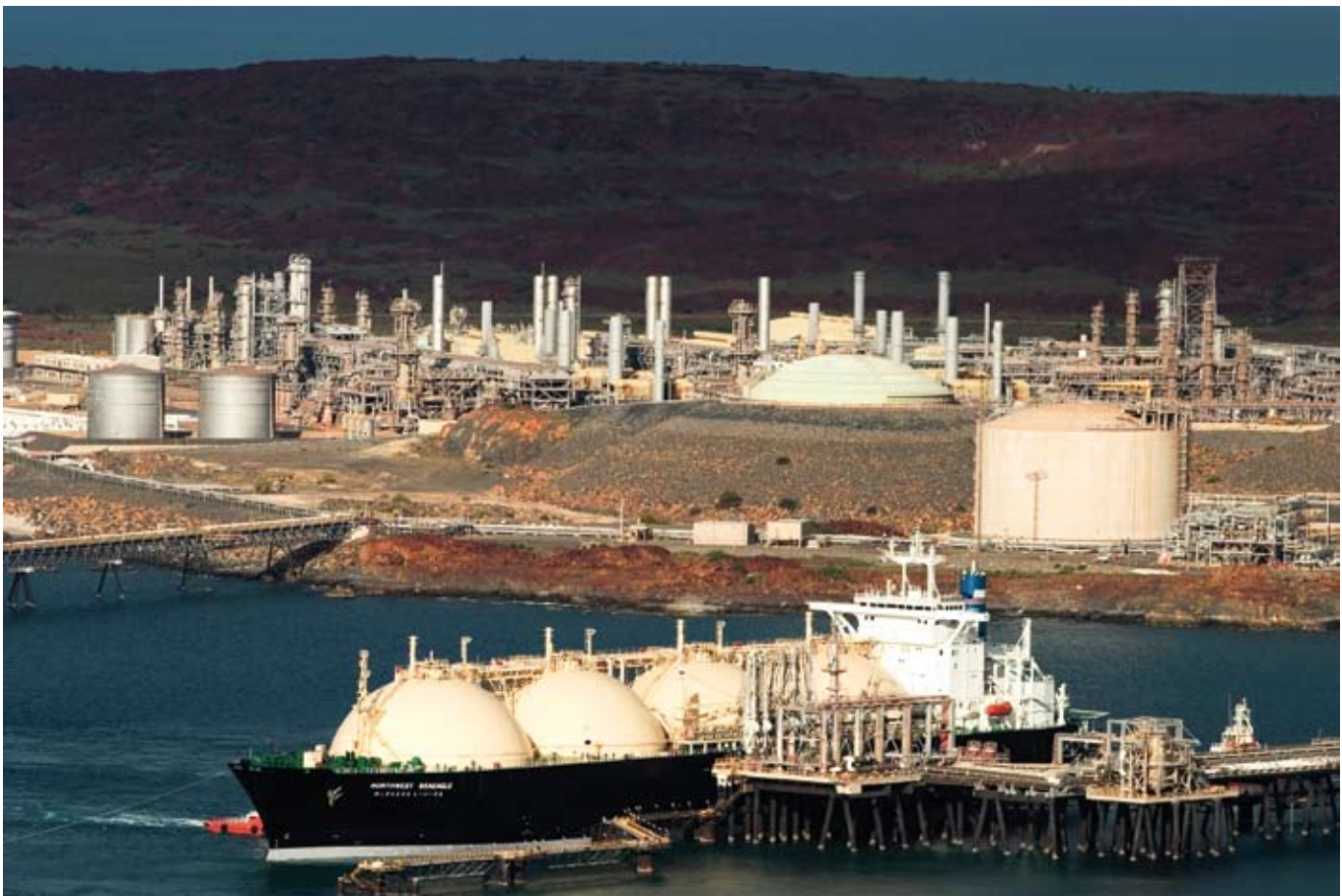
Woodside's Karratha Gas Plant, North West Shelf Venture, Western Australia © Woodside
